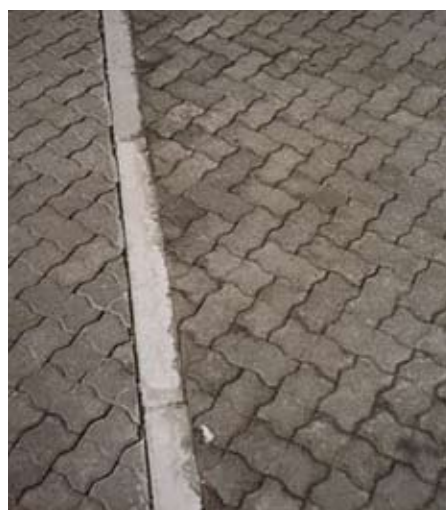
Photograph 1 – Anchor beam, showing gap due to creep of blocks immediately downside of anchor beam
